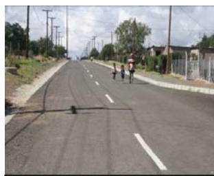
L Section: Bot Rd 551 – Project completed
