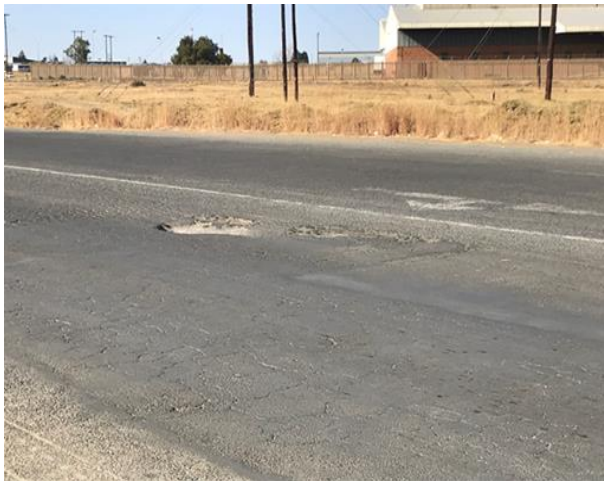
Figure 7: Potholes identified of Kgosimang Dimpane Street
