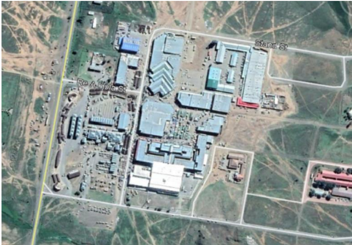
Figure 7.3: Botshabelo transfer facility
